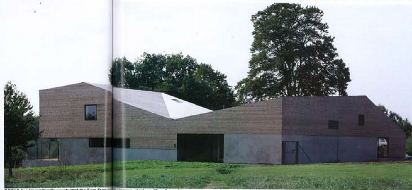
DSDHA has intermittently punctuated the Sure Start with windows, playing with notions of transparency and privacy.
