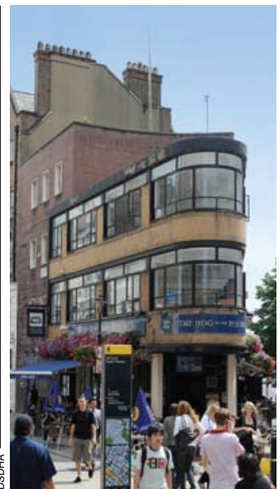
Above Aerial view down South Molton Street with HMV building now occupied by Foot Locker Far right The 'prow' is conceived as thrusting into the path of Oxford Street's hordes of shoppers Centre right Junction with no 27 South Molton Street Right The demolished pub
