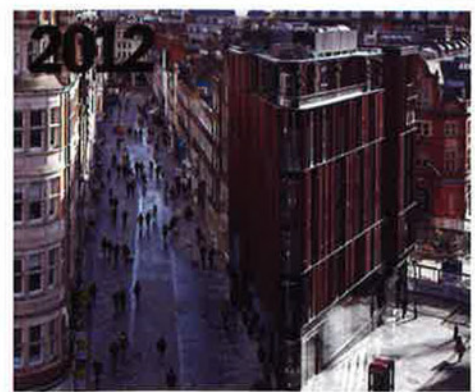
2012 South Moulton Street Building, London W1 DSDHA
