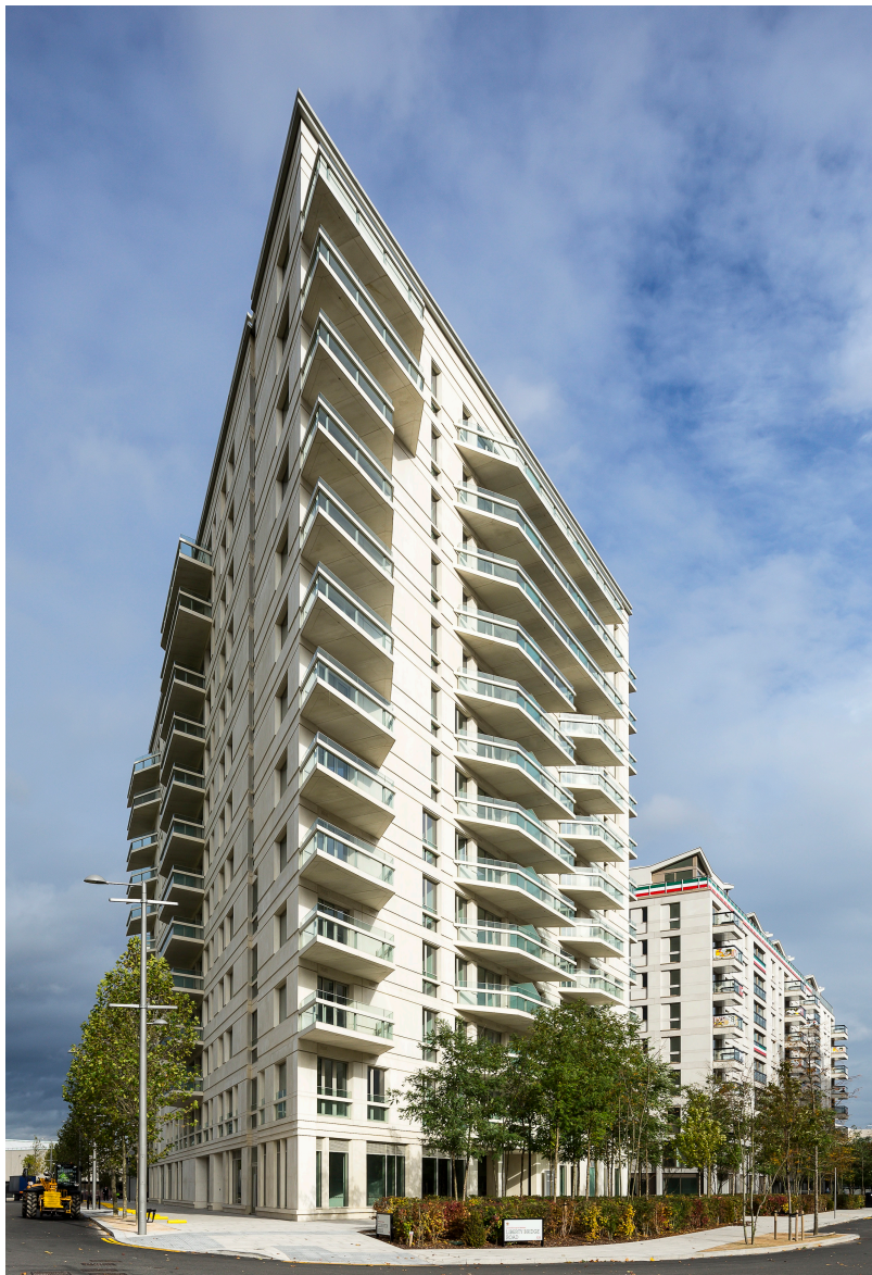
Fig. 1. Main approach view of Vesta House
