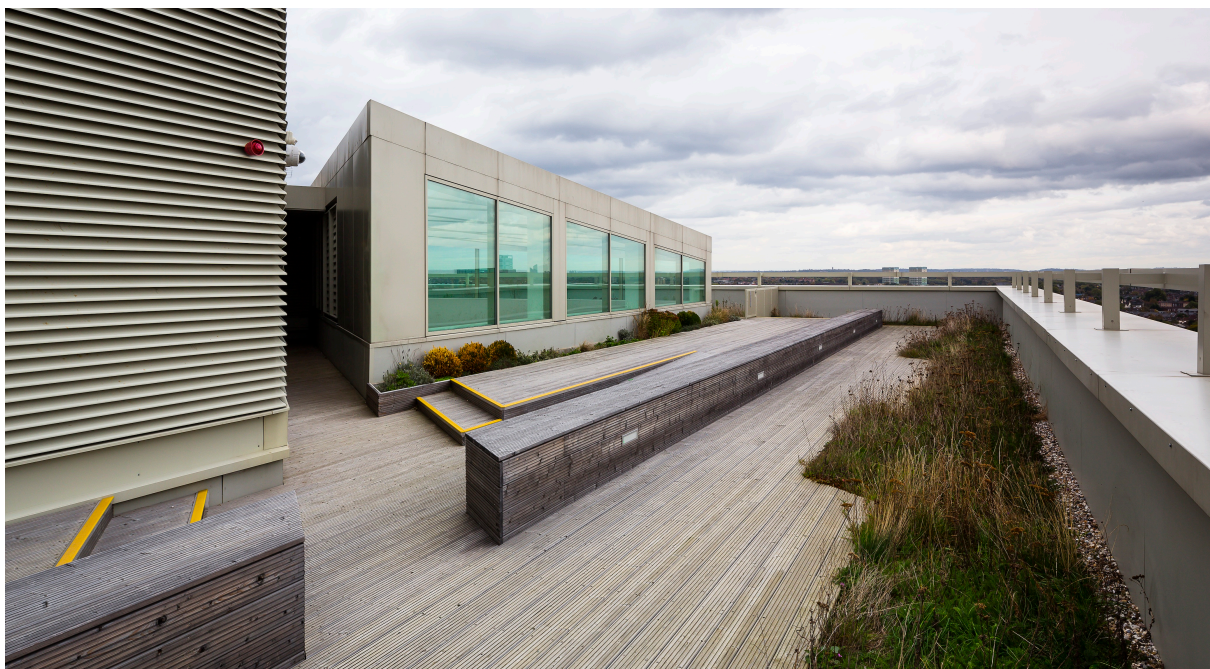
Fig. 13. Roof top terrace, photography by Dennis Gilbert
